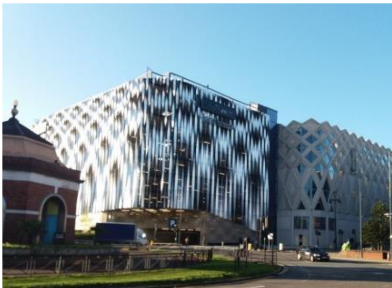
Figure 2.25 Leeds Shopping Centre Car Park
